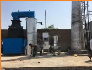
Thermic Fluid Heater
