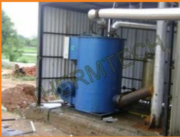
Vertical Hot Water Generator
